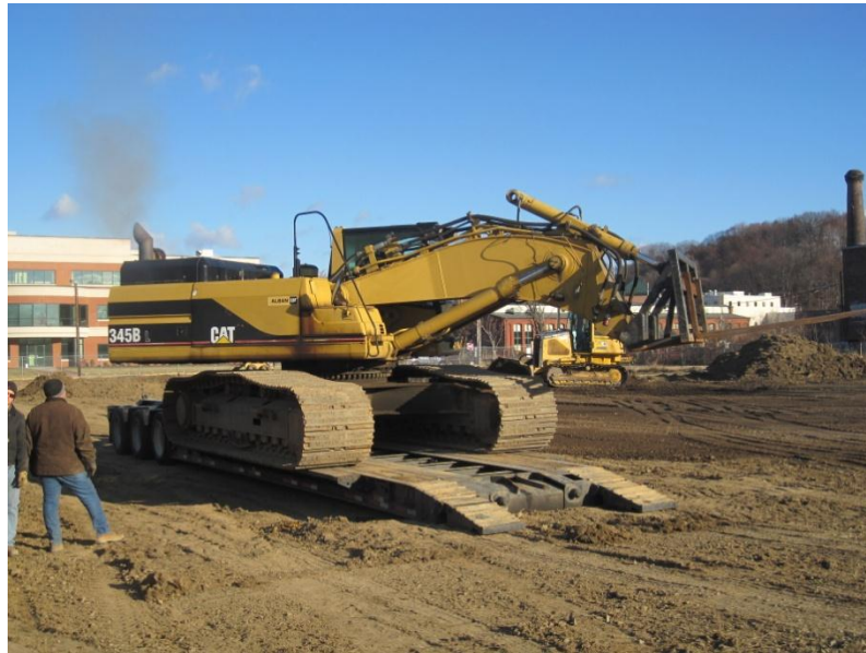
Figure 54. Mobilization of hydraulic excavator
