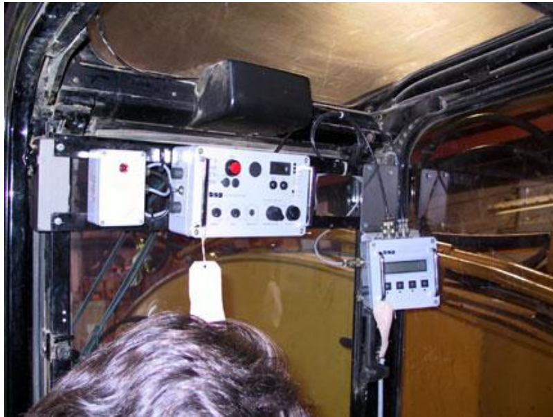
Figure 4. RIC data acquisition system (from Rapid Impact Compactors, Ltd 2004)
