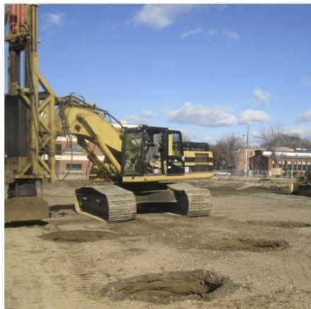
Rapid Impact Compactor following first pass of compaction points
