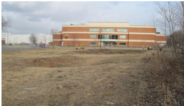
Figure 60. Depression on site prior to backfilling
